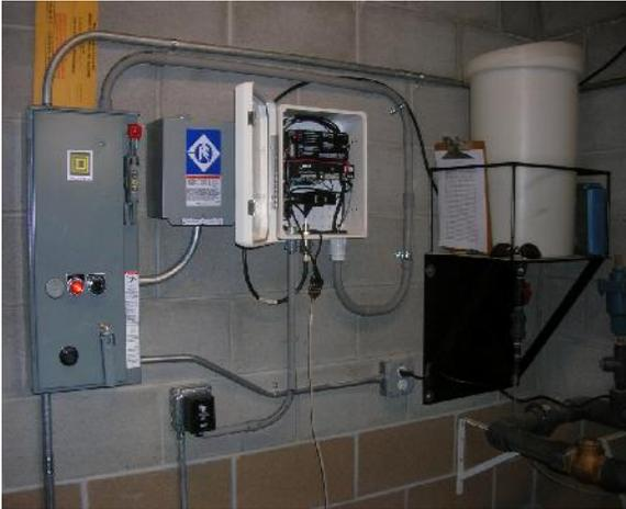
When the management building at the entrance to the State Park was completed, we installed a Base Station, which consisted of an RF401 Spread Spectrum Radio with a small Dipole antenna. The RF401 is connected to a local desktop PC. The PC is running LoggerNet software. The Park Service personnel can see what the current tank water level is and if they need to, they can turn on or off the pump in the pump building remotely, without leaving their office.
