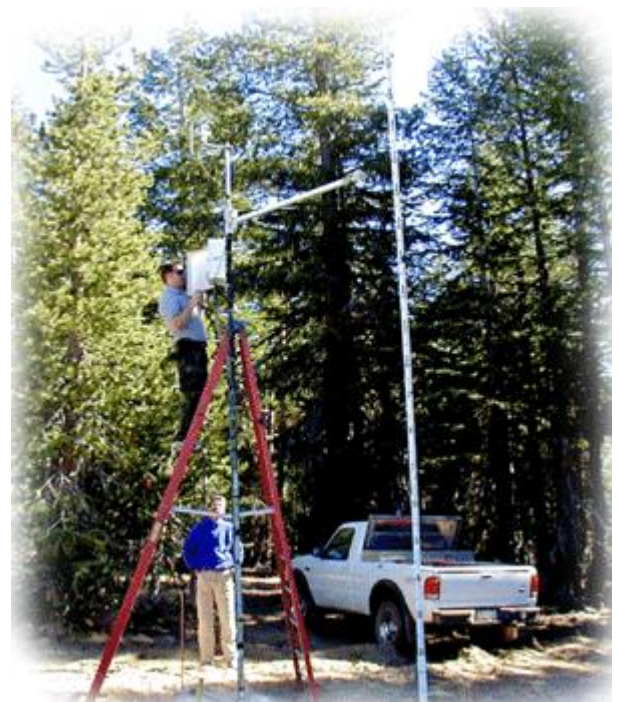
Intermountain Environmental personnel complete final installation and testing at the upper site.
