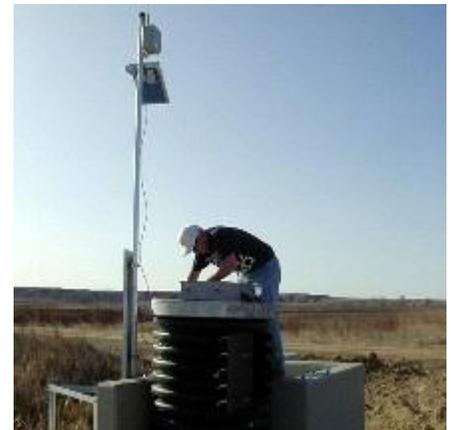
*IEI personnel installing remote water level monitoring system at Sheppards Bottoms site*
