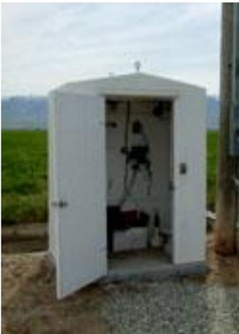
*Fiberglass Instrument Shelter at the Lower Diversion. This shelter house the Measurement and Control Unit and power supply.*
