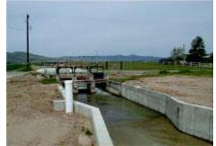
*Lower Diversion. Bear River water enters from the top, Cub River water enters from the right, and the combined water is then diverted to canals on the left and bottom. The white PVC pipe on the left of the canal houses an ultrasonic distance sensor.*
