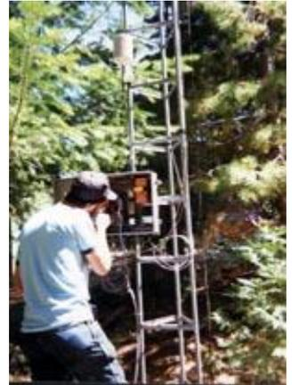
*Weather Station being installed on 130 ft. Triangular Instrument Tower*
