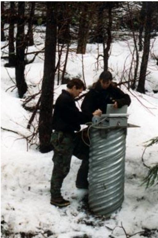
*R2 Data logger with attached FP10C Float & Pulley Sensor being installed on stilling well by a stream at Blodgett Forest Research Station.*
