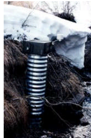
Large military ammunition canister mounted to a corrugated pipe to make a still well and instrument plat form.
